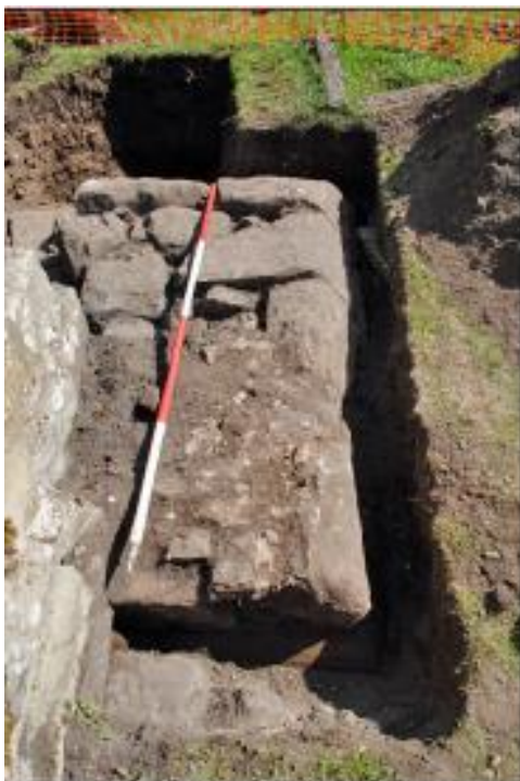
Illus. 46: View looking south across completed excavation of Tower foundations adjacent to the southwest corner of the Nave.
