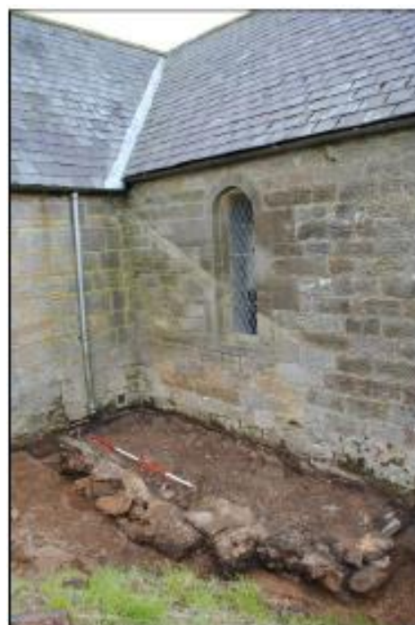
Illus. 22: View looking southeast at structural remains at intersection of the north transept and north nave wall.
