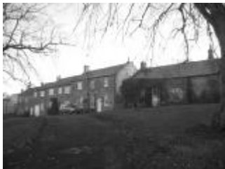
A picture taken in 2005 of the premises of the former Dixon's Shop, with Rose Cottage on the right and the former shop warehouse on the left.
